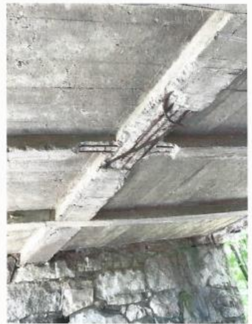
Bridge Underside showing concrete deterioration
