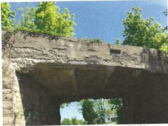
Closeup showing concrete deterioration, looking north.
