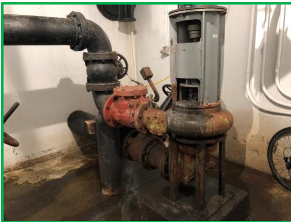
One of the Lift Pumps at Village WWTP (photo credit Zachary Johnson)
