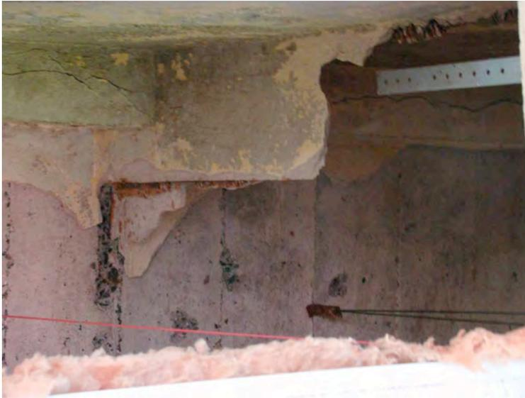
Loss of plaster on concrete ceiling.
