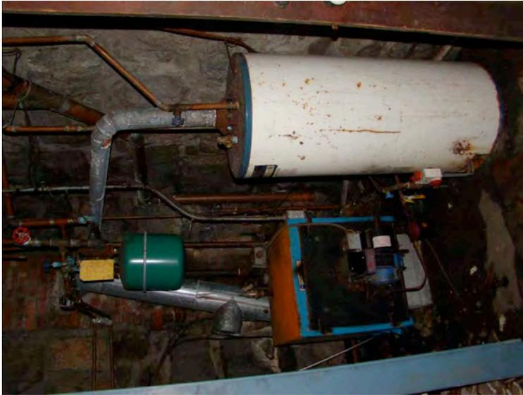
Boiler & hot water tank in basement. Neither has been used for several years.
