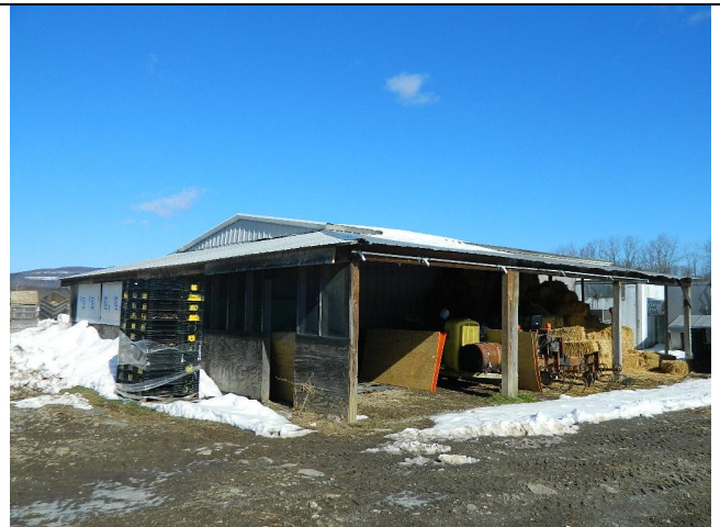
Utility barn (south & east side views)
