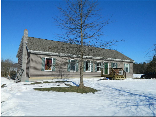
Front view of dwelling
