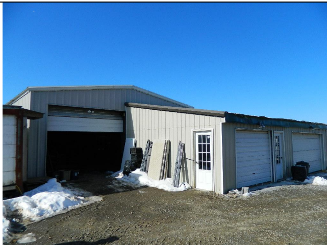
Utility barn (north side view)
