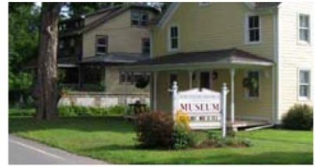
The traditional detailing of this sign is in keeping with the architectural style of the building, and it is tastefully landscaped.
