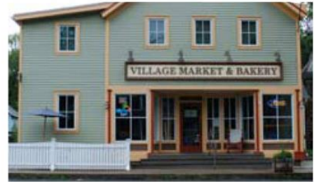
This highly legible sign is perfectly designed to match the character of the building facade, and downlighting prevents glare and light pollution.
