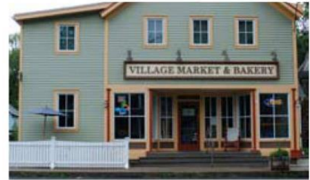
This highly legible sign is perfectly designed to match the character of the building facade, and downlighting prevents glare and light pollution.
