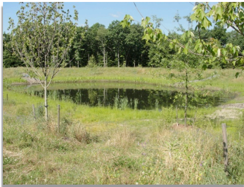
Detention Pond for Drainage at Woodland Pond
