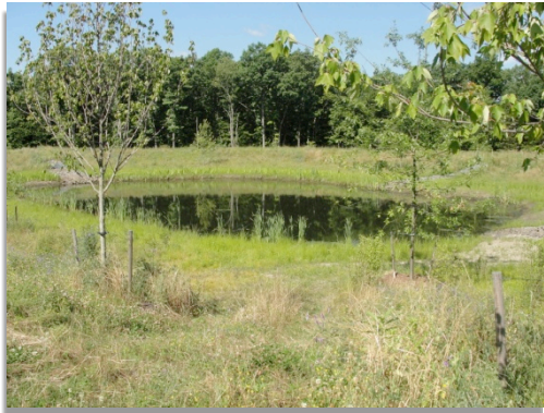
Detention Pond for Drainage at Woodland Pond
