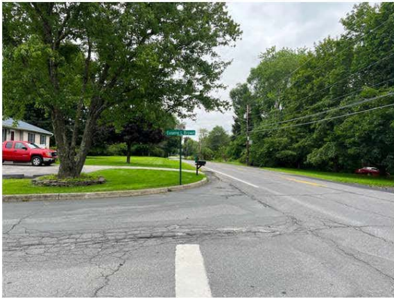
3. Facing North on Route 32
