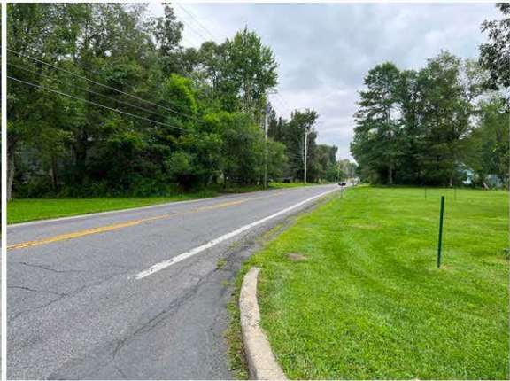
4. Facing South on Route 32
