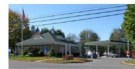
A drop-off area in Brewster, New York, uses a clear island, the site of the entrance to the large driveway to the parking area and landscaping, as well as a sign placement and landscaping to separate the road from the parking area.
