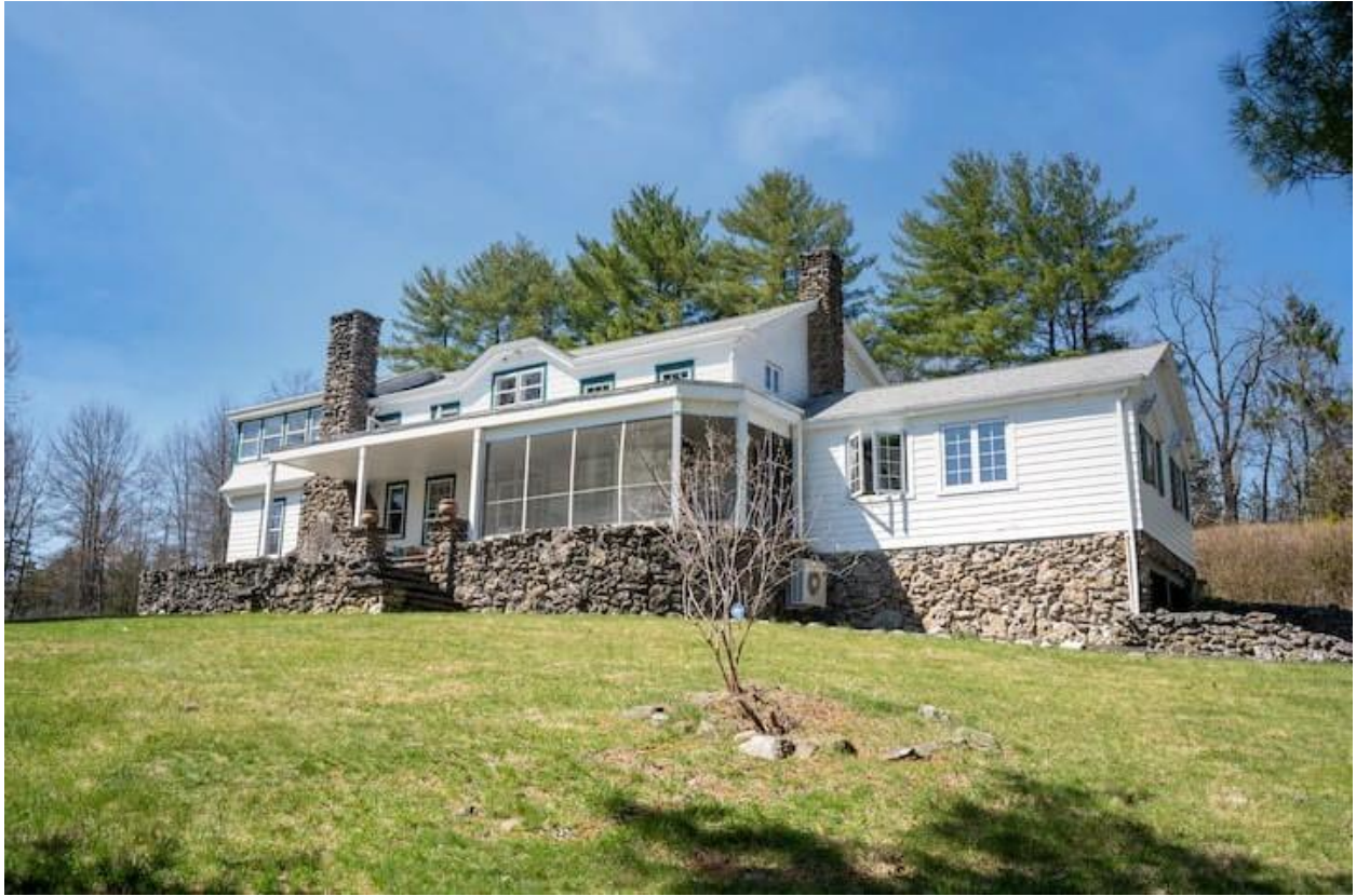
Image 6- Main house, Front (west) and side (south) elevations. Note the garage doors present on the side elevation, which connects to the blacktop driveway.
