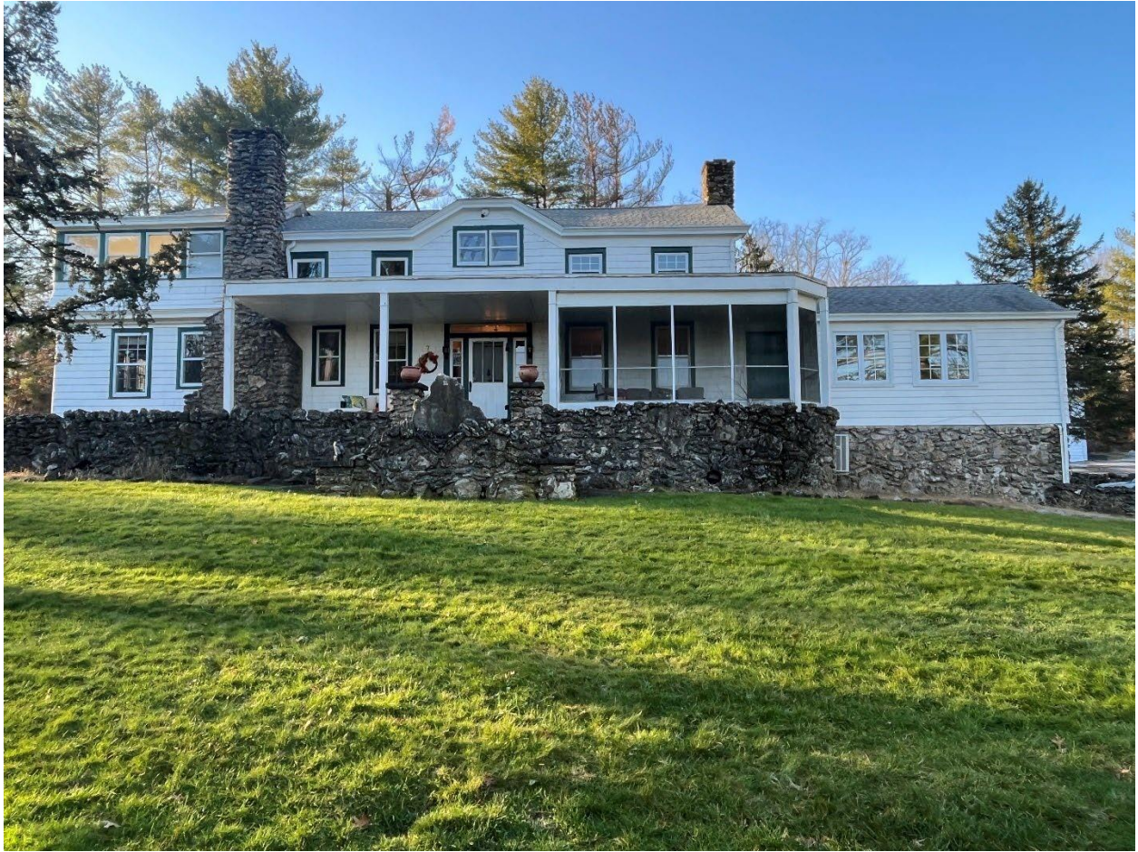
Image 5 -Main House, front (west) elevation showing prominent stone base and entryway.
