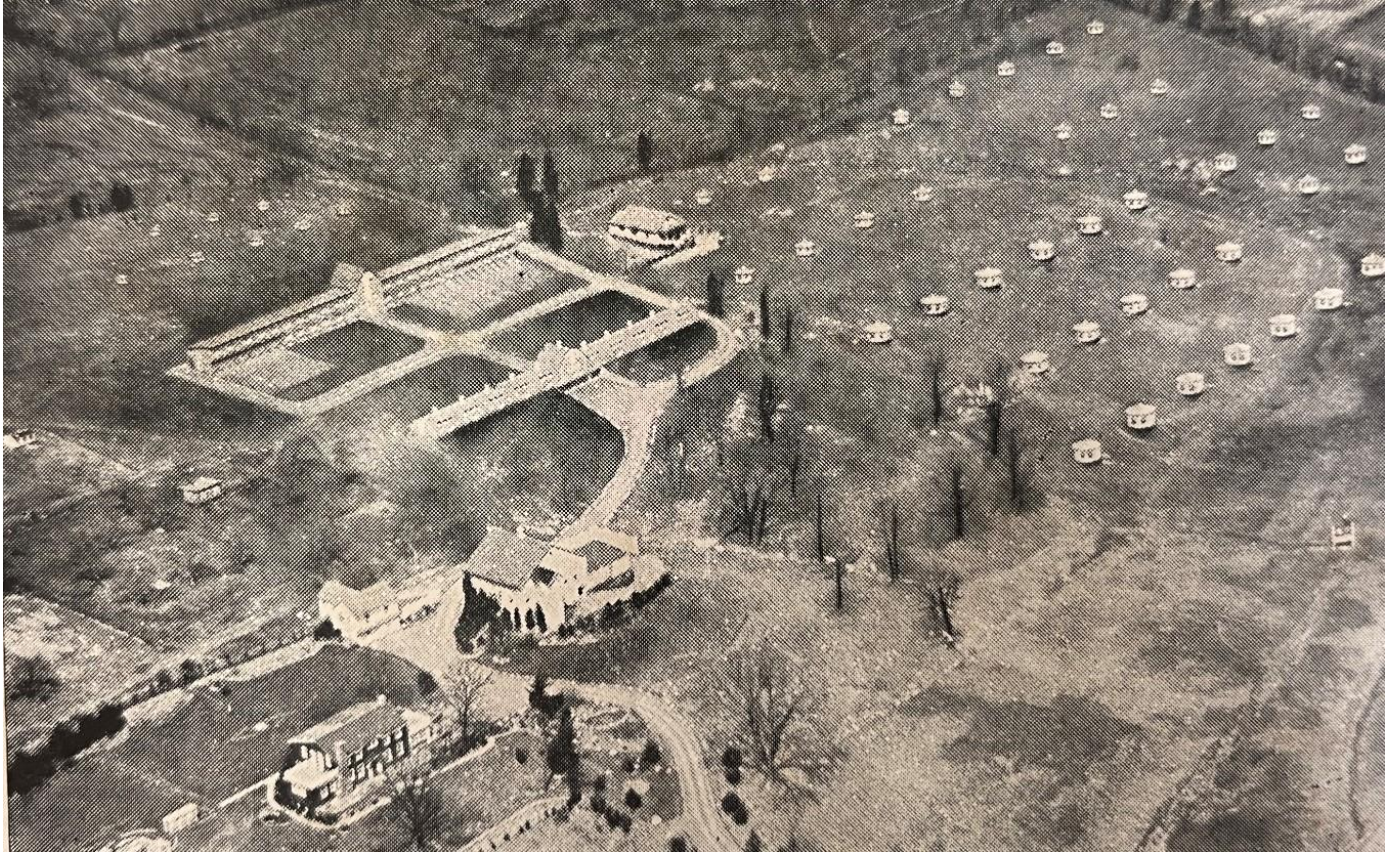
Image 25– Ca. 1939 Aerial Photograph of the Kauder Chicken Farm, over 30 years before the property was purchased by Patterson. Note the presence of the three main buildings by this point in time, as well as the additional outbuildings which are no longer extant.
