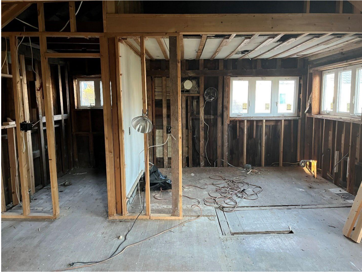
Image 21- Cottage, Interior looking north at unfinished interior.
