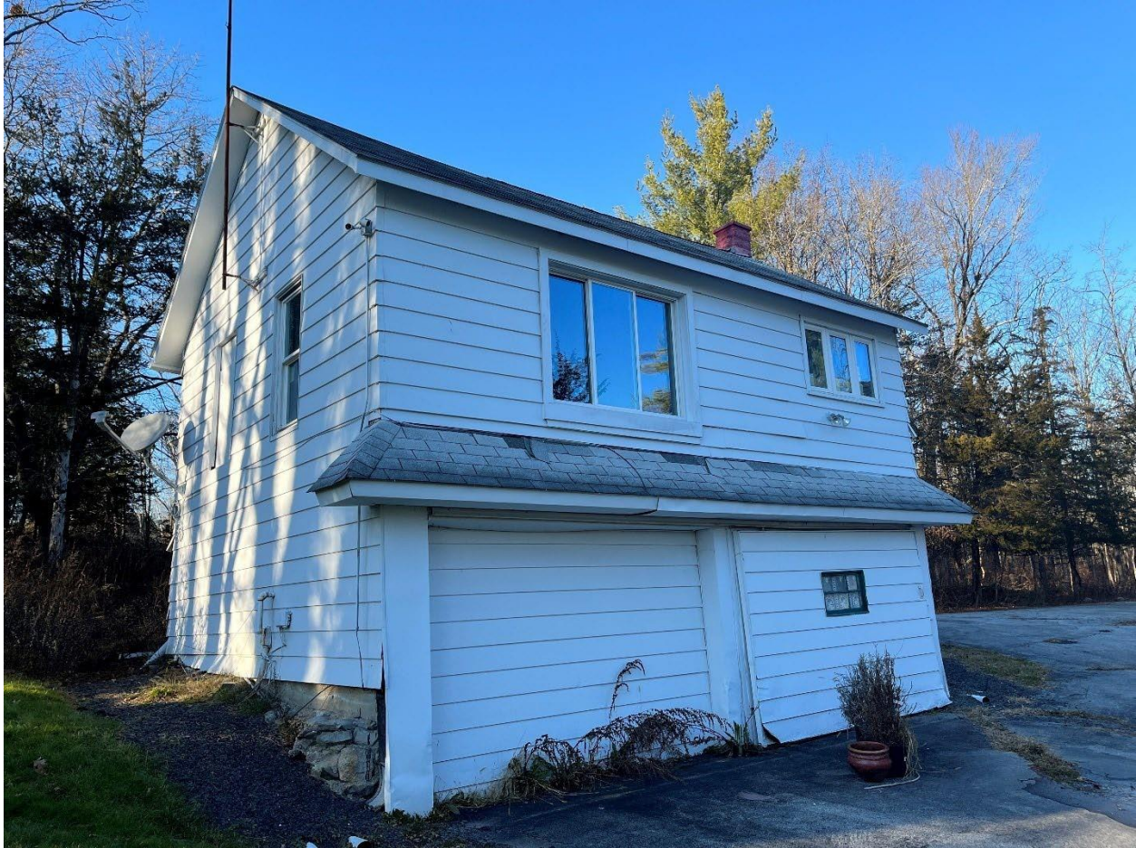
Image 20- Cottage, Side (south) and rear (west) elevations facing blacktop driveway.
