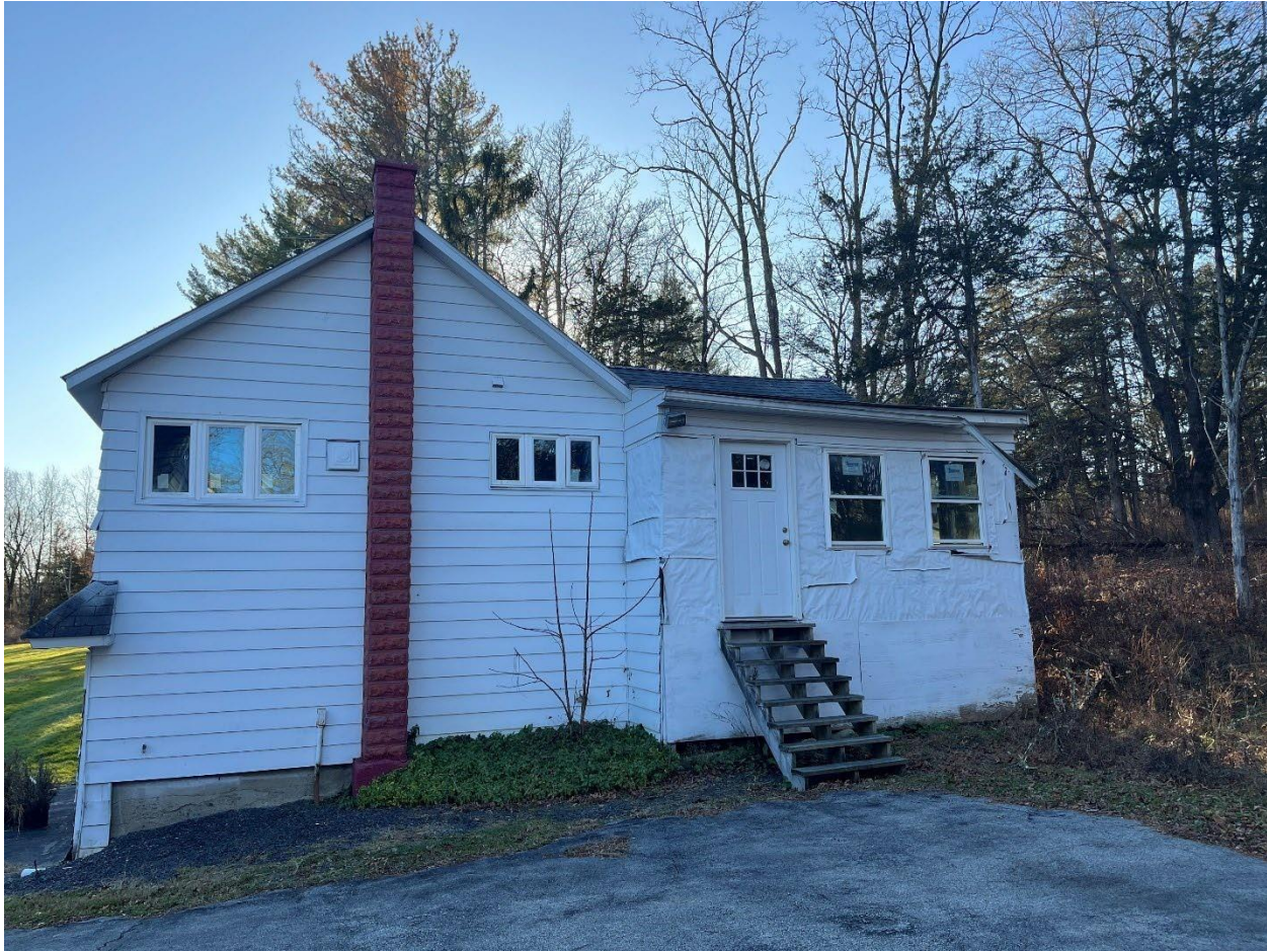
Image 19- Cottage, Front (east) façade showing the primary entrance to the building.
